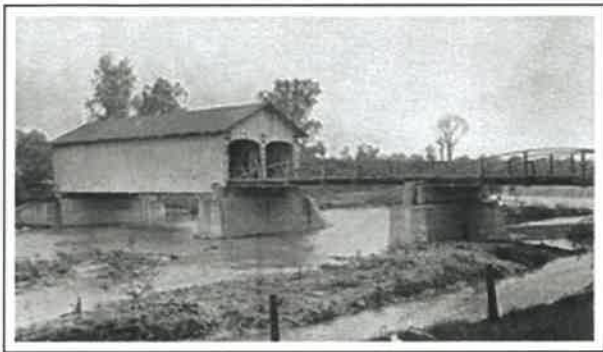
Main Street crossed the Huron River via a covered bridge built in 1836-1837. The landmark bridge was far too frail to support interurban cars and was replaced in 1910.
